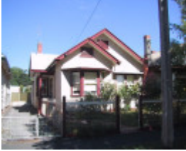
224 Raglan Street South
