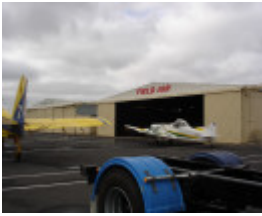
14247 Former Ballarat RAAF base Bellman Hangars
