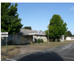
FORMER BALLARAT RAAF BASE SOHE 2008
