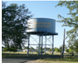
FORMER BALLARAT RAAF BASE SOHE 2008
