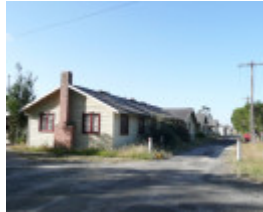
FORMER BALLARAT RAAF BASE SOHE 2008
