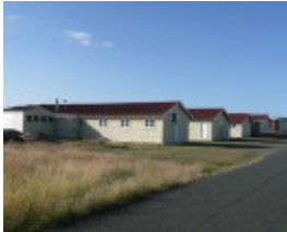
FORMER BALLARAT RAAF BASE SOHE 2008
