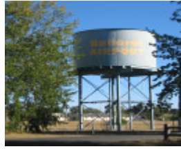
14247 Former Ballarat RAAF Base water tower
