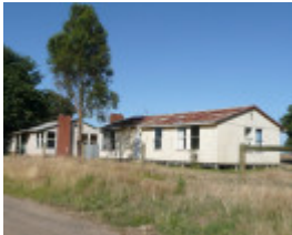
FORMER BALLARAT RAAF BASE SOHE 2008
