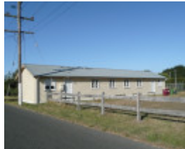
FORMER BALLARAT RAAF BASE SOHE 2008
