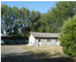
FORMER BALLARAT RAAF BASE SOHE 2008
