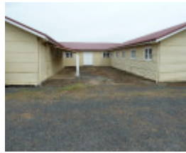
H2113 FORMER BALLARAT RAAF BASE LHA 2015 4.JPG
