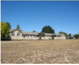
14247 Former Ballarat RAAF Base Admin building
