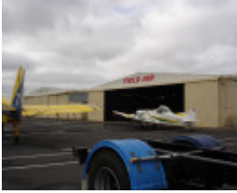
14247 Former Ballarat RAAF base Bellman Hangars
