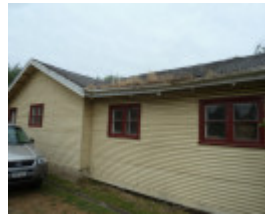
H2113 FORMER BALLARAT RAAF BASE LHA 2015 3.JPG
