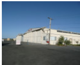
FORMER BALLARAT RAAF BASE SOHE 2008
