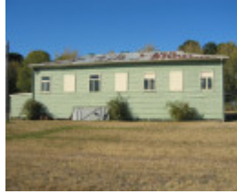
14247 Former Ballarat RAAF Base gymnasium
