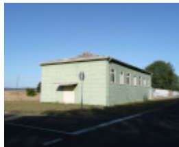
FORMER BALLARAT RAAF BASE SOHE 2008
