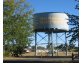
14247 Former Ballarat RAAF Base water tower
