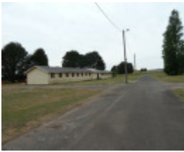
H2113 FORMER BALLARAT RAAF BASE LHA 2015 2.JPG
