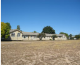
14247 Former Ballarat RAAF Base Admin building
