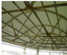
14252 Hamilton racecourse 4Sept06 grandstand roof
