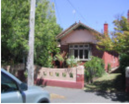
24 Raglan Street South
