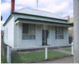
220 Peel Street North
