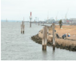
Newport Pier Williamstown Aug 2003 Timber Dolphins And Stone Embankments
