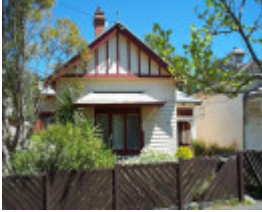
329 Lydiard Street North
