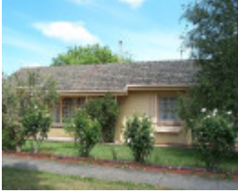
807 Lydiard Street North
