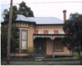
207 Peel Street North
