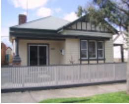
230 Peel Street North
