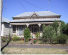
216 Raglan Street South
