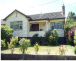
802 Lydiard Street North
