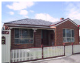
234 Peel Street North
