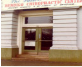
former bank of nsw view street bendigo entrance
