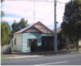
323 Peel Street North
