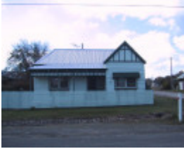
18 Otway Street North
