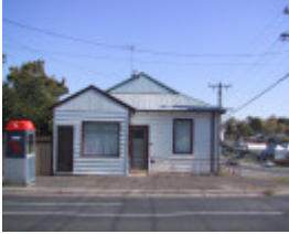
421 Peel Street North
