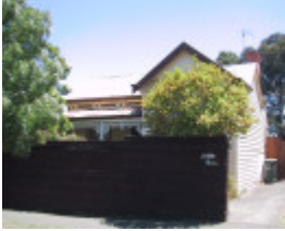
414 Raglan Street South
