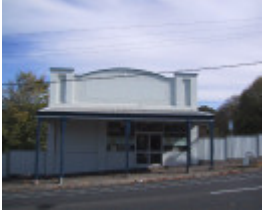
331 Peel Street North
