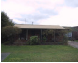
202 Peel Street North
