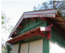
Gable detail. Mar 2007
