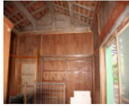
General internal view. Mar 2007.
