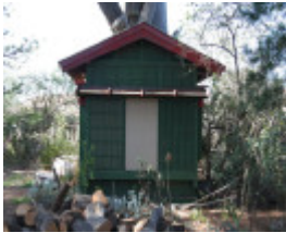
General external view. Mar 2007.
