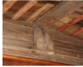
Gable end structure - internal view. Mar 2007.
