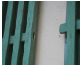
Lattice detail. Mar 2007.
