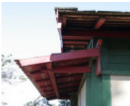
Eaves detail. Mar 2007.
