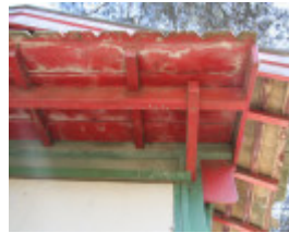
Eaves detail. Mar 2007.
