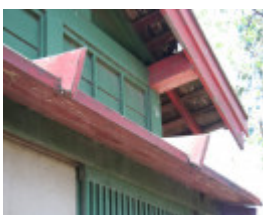
Roof detail. Mar 2007.
