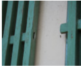
Lattice detail. Mar 2007.
