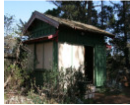
General external view. Mar 2007.
