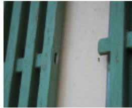
Lattice detail. Mar 2007.
