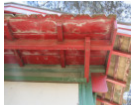
Eaves detail. Mar 2007.
