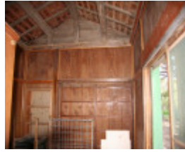
General internal view. Mar 2007.
