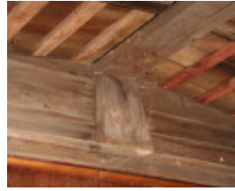
Gable end structure - internal view. Mar 2007.
