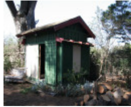
General external view. Mar 2007.
