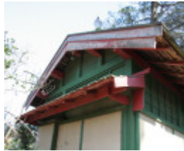
Gable detail. Mar 2007
