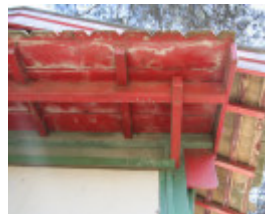
Eaves detail. Mar 2007.
