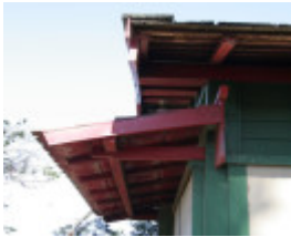
Eaves detail. Mar 2007.
