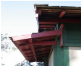
Eaves detail. Mar 2007.
