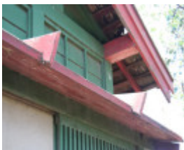
Roof detail. Mar 2007.
