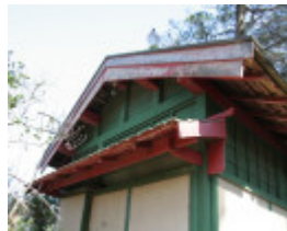
Gable detail. Mar 2007
