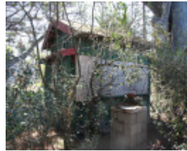
General external view. Mar 2007.
