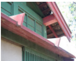
Roof detail. Mar 2007.
