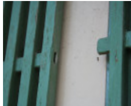
Lattice detail. Mar 2007.
