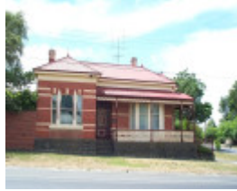
402 Lydiard Street North
