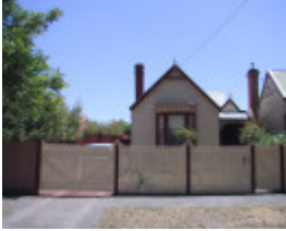
328 Raglan Street South
