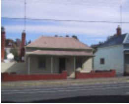
313 Peel Street North
