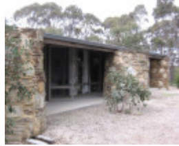
H2118 Baker House Bacchus Marsh west elevation rc May 2006
