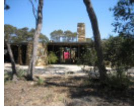
H2118 Baker House Bacchus Marsh Ext Facade Dec 2006 mz
