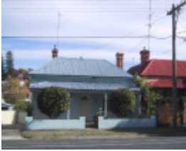
315 Peel Street North
