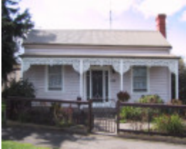
228 Peel Street North
