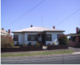
415 Peel Street North
