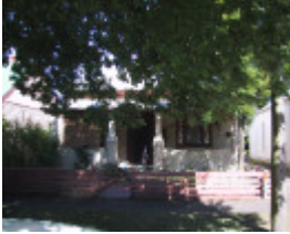
124 Raglan Street South
