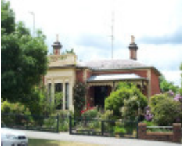
330 Lydiard Street North
