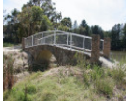
H0398 Callembeen Pk 14 Feb 07 PM2 Footbridge
