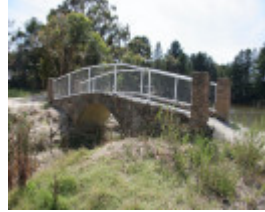
H0398 Callembeen Pk 14 Feb 07 PM2 Footbridge
