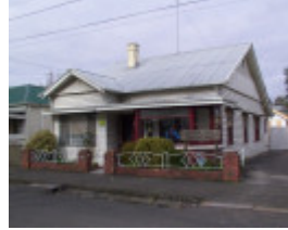
36 Steinfeld Street South
