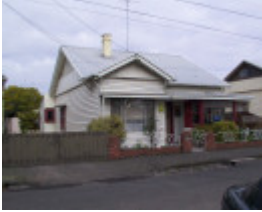
36 Steinfeld Street South
