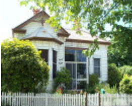
602 Lydiard Street North
