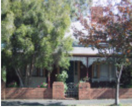
419 Peel Street North
