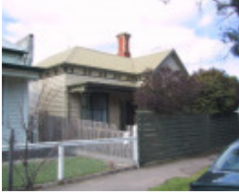
218 Peel Street North
