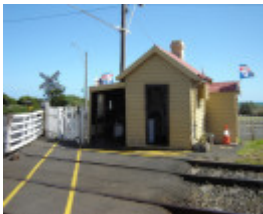
Gatekeepers cabin Railway Gates New Street Brighton Nov 2006
