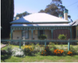
611 Ripon Street South
