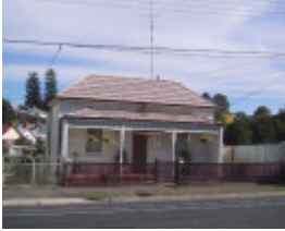
309 Peel Street North
