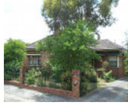
514 Lydiard Street North
