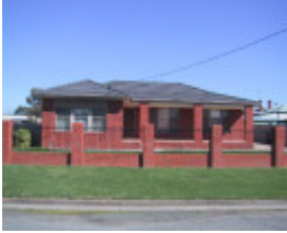
23 King Street North
