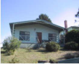
409 Peel Street North
