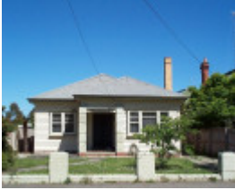
807 Armstrong Street North
