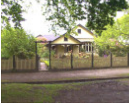
9-9a overall view Carlton Street
