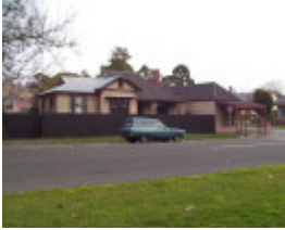
701- side view from gladstone street Barkly Street
