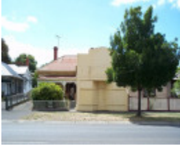
618 Lydiard Street North
