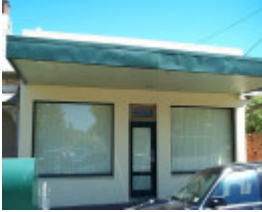
313 Lydiard Street North
