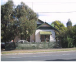
319 Peel Street North
