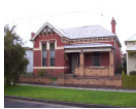
35 Anderson Street East
