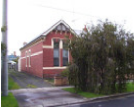
35 Anderson Street East
