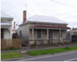
58 Peel Street South
