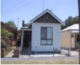
322 Raglan Street South
